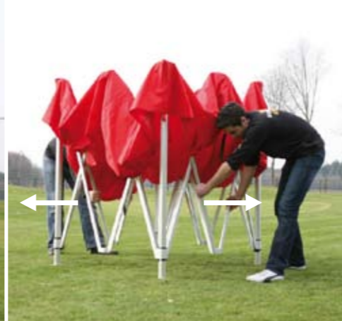
STEP 3 PULL THE FOLDING TENT OPEN FROM BOTH SIDES, UNTIL THE FOOTPRINT SIZE HAS BEEN REACHED
